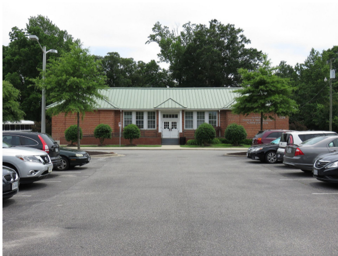
East Suffolk Elementary School
